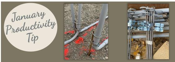
Conner Webber shared an idea he seen on a project of how the electricians use fabbed brackets to speed up ground work process. This type of thinking could help us in the future for securing water piping.
